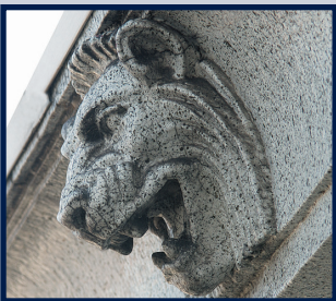
Details from the columns outside of the building.
